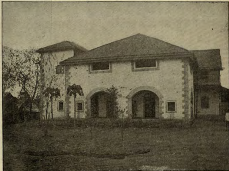
Mission Building, Igatpuri, India
